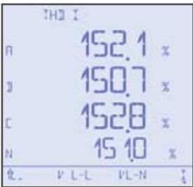
Current total harmonic distortion display
